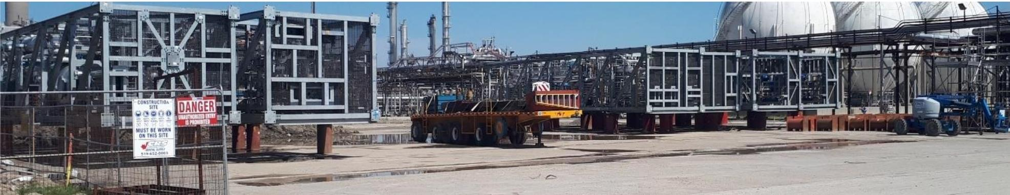
Core process modules awaiting installation
